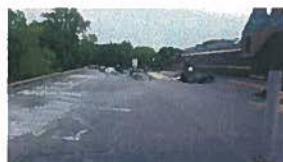
Flat Roofing Replacement
