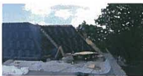
Slate Roofing Removal
