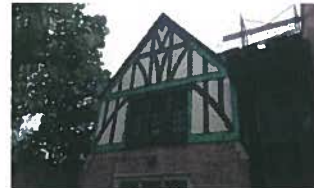
Gable End Wood Trim Replacement
