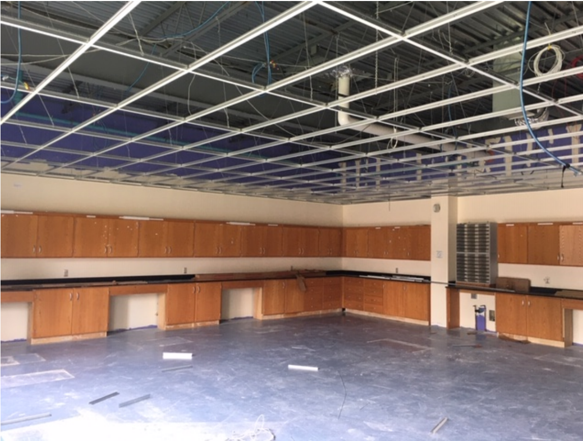
Week 9 – Installing new ceiling grid for support of new ceiling tiles and new light fixtures in an existing Classroom in the Science Wing
