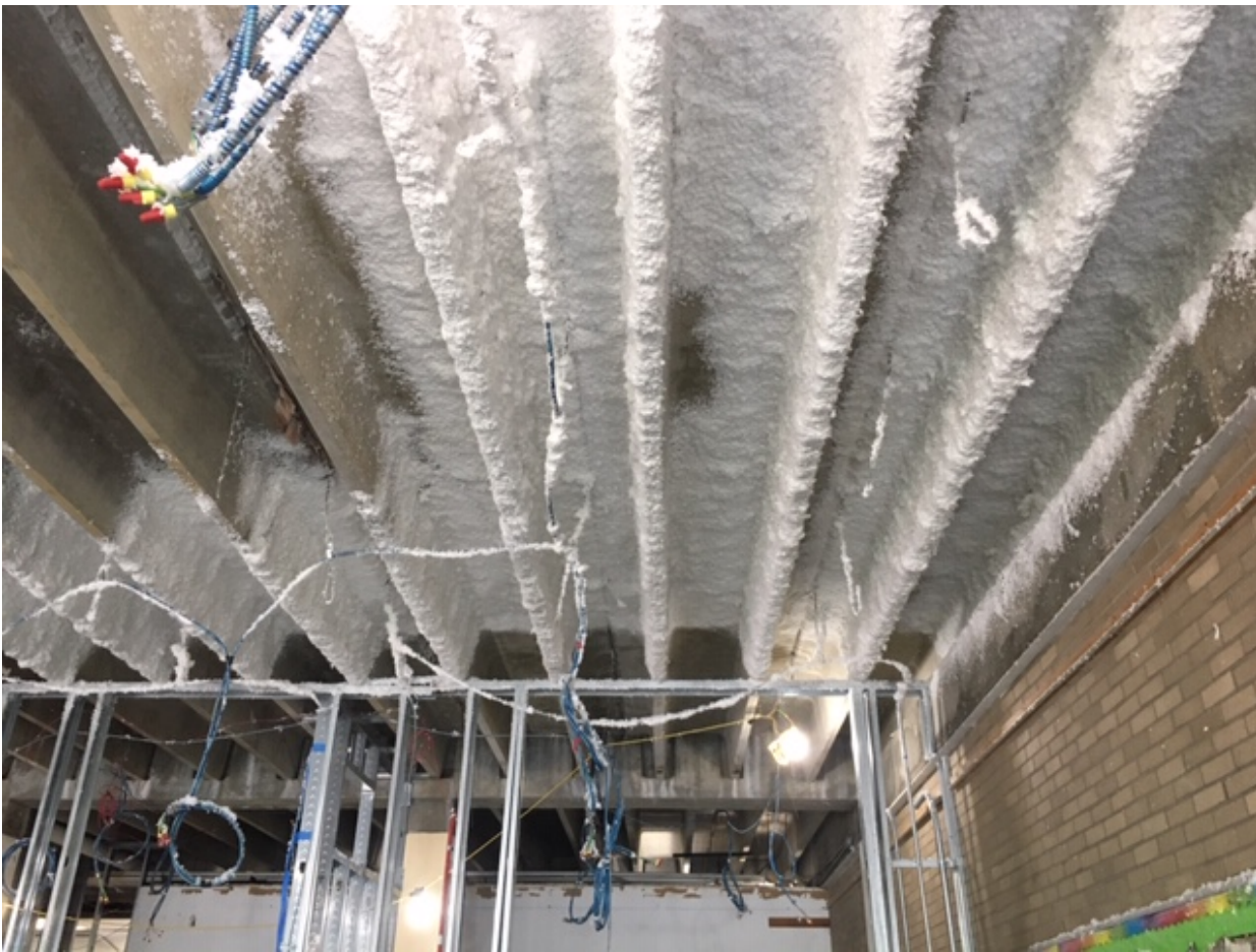
Week 9 – Spraying acoustical foam material onto the underside of the existing deck in the Music Wing
