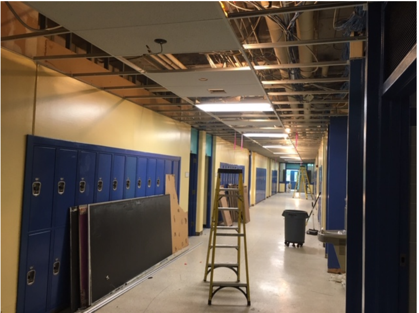
Week 9 – Installation of ceiling grid & light fixtures in Classroom Corridor
