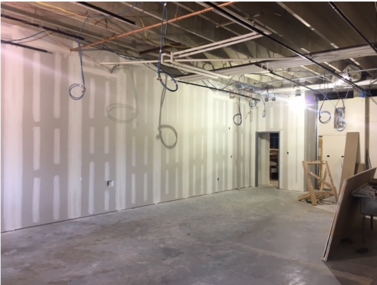
Week 9 – Partition in Art Wing Classroom ready for priming & painting
