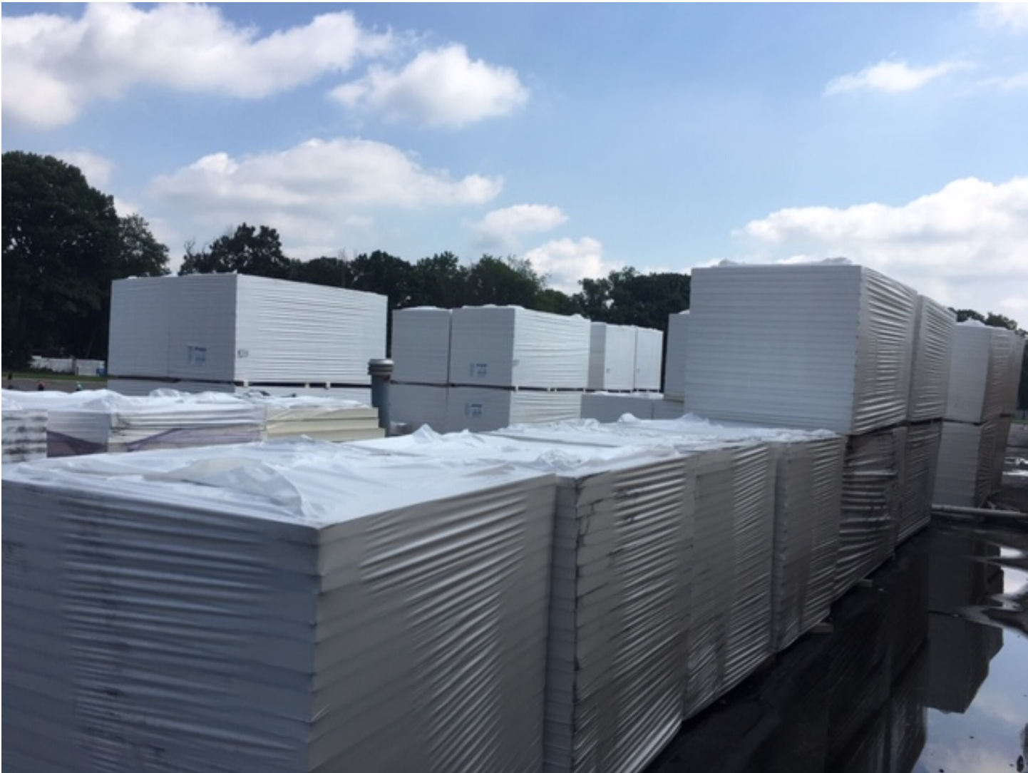
Week 9 – Staging of material for the installation of the new roof assembly over the Locker Rooms
